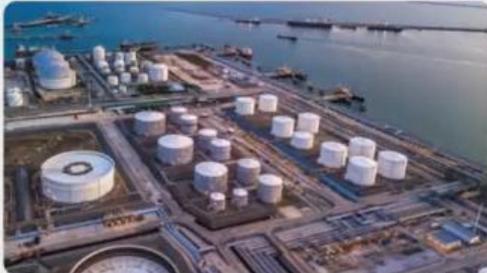
Soil-side corrosion of aboveground storage tank (AST) bottoms is a major challenge. ASTs typically include active cathodic protection (CP) systems to mitigate this corrosion.
